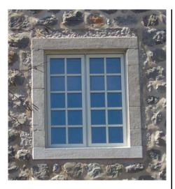
SDL (Simulated Divided Lites) refers to windows with fully-profiled muntins that cover both sides of a thermal glass panel to create the effect of a series of smaller window panes. Generally, SDLs should include spacer bars in between the muntins within the thermal glass.
